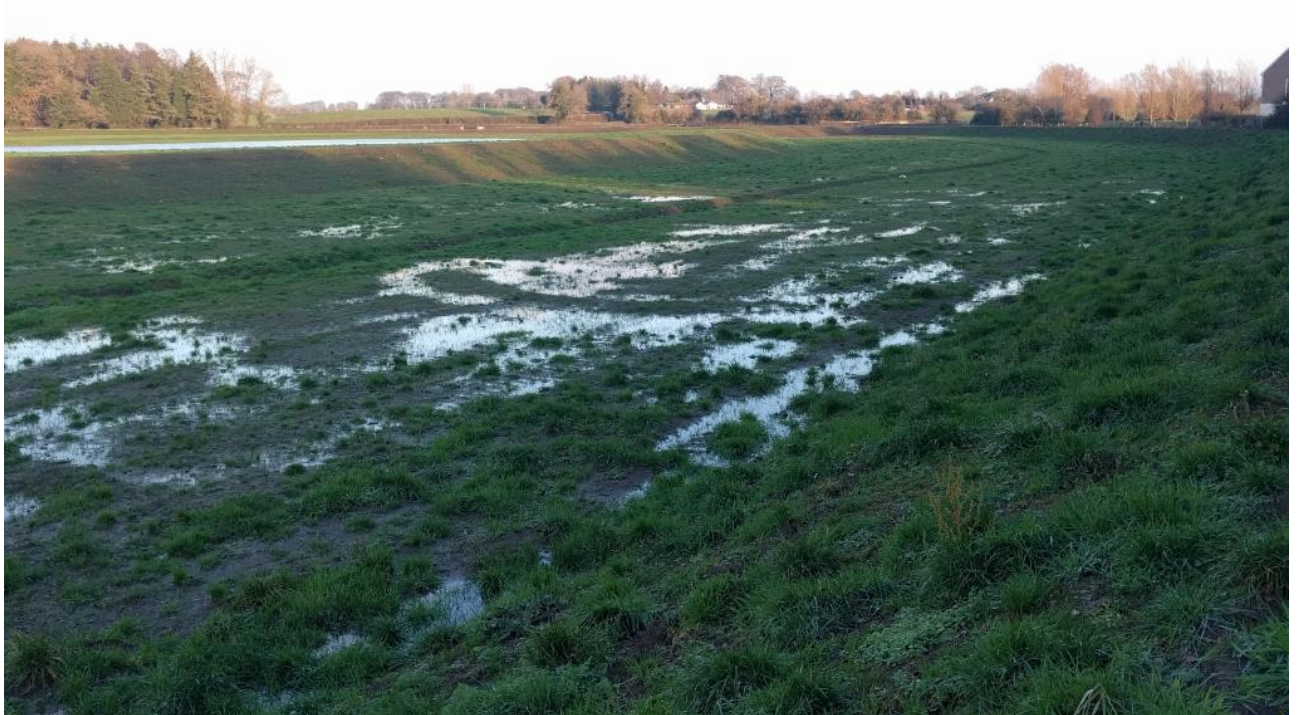
Photo 10 – Completed 'Upper Ditch' Flood Plain Works
