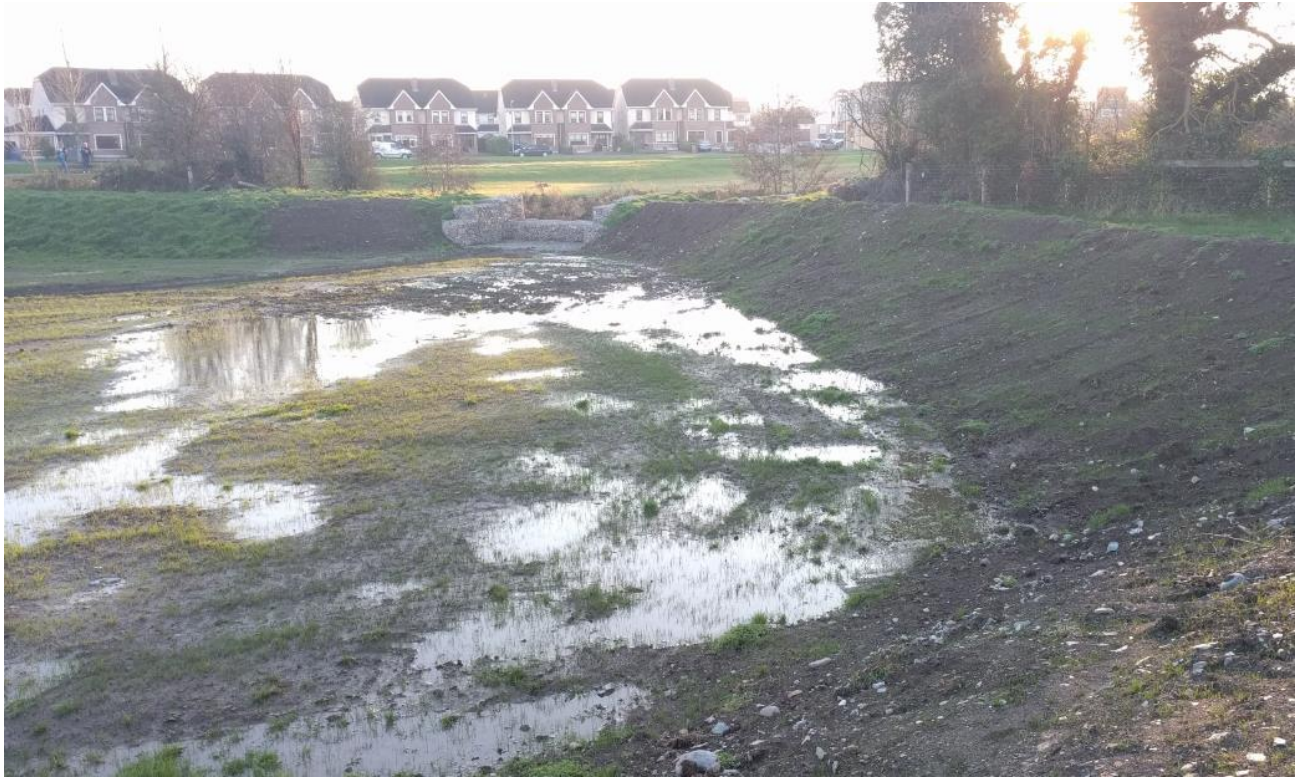
Photo 9 – Completed 'Upper Ditch' Flood Plain Works
