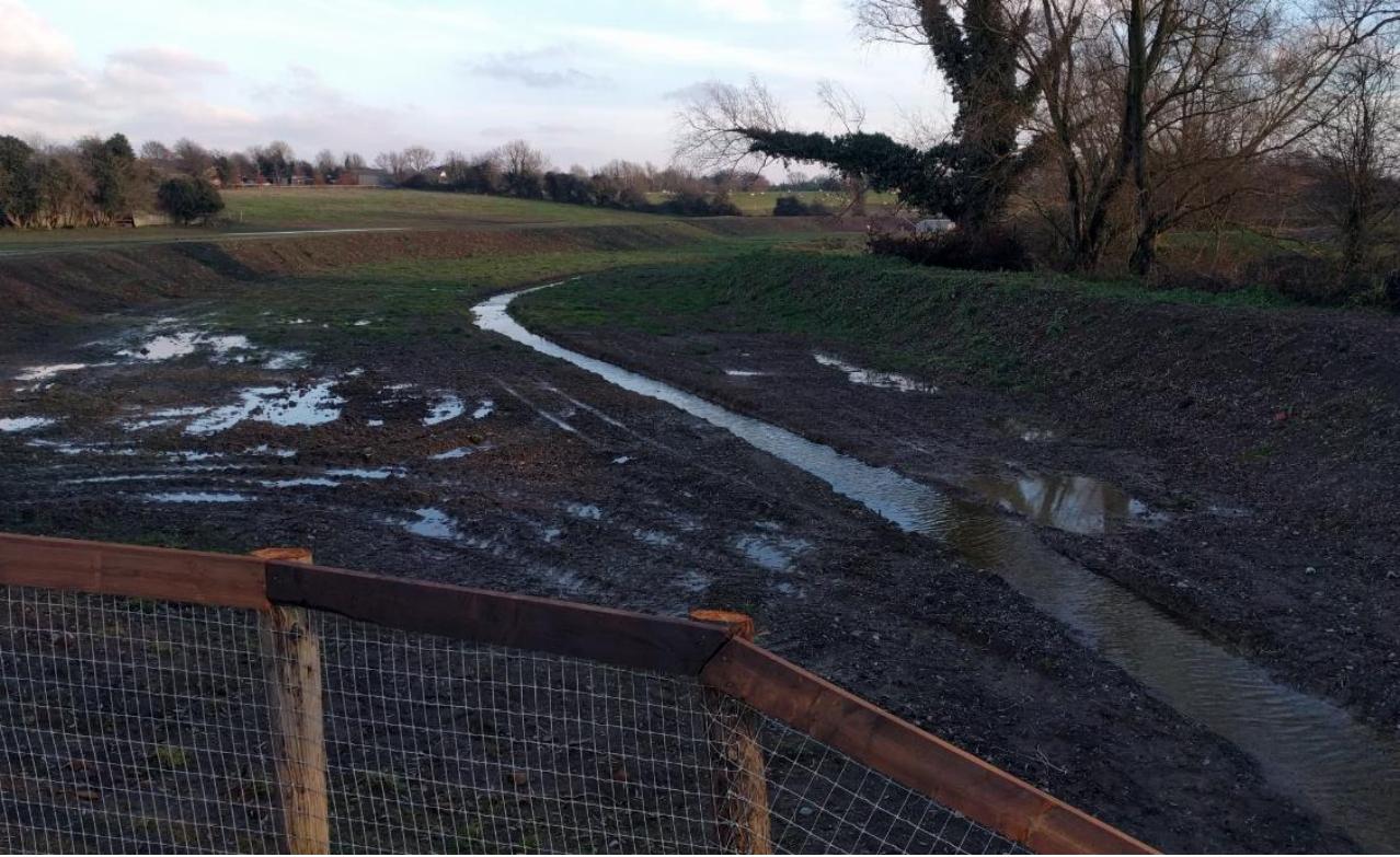
Photo 7 – Completed 'Upper Ditch' Flood Plain Works
