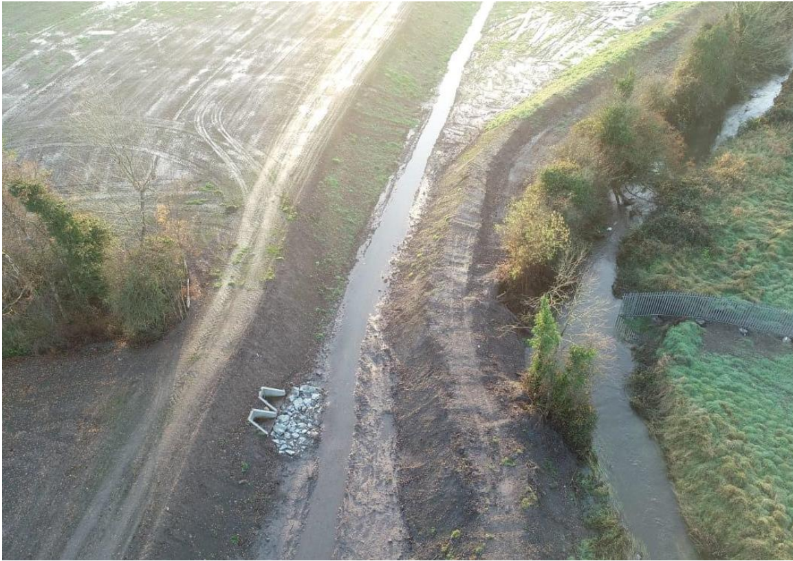
Photo 4 – Completed 'Upper Ditch' Flood Plain Works
