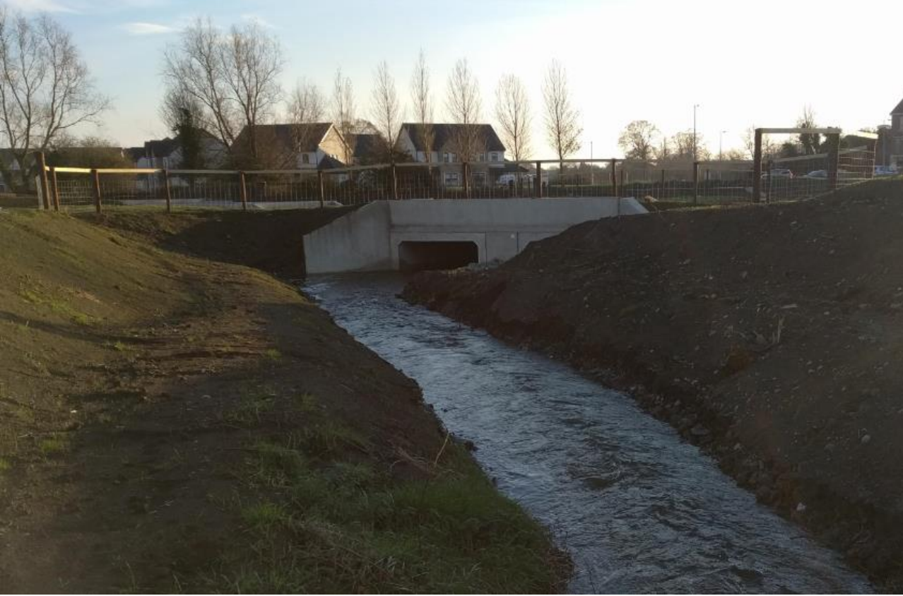
Photo 8 – Completed 'Upper Ditch' Flood Plain Works
