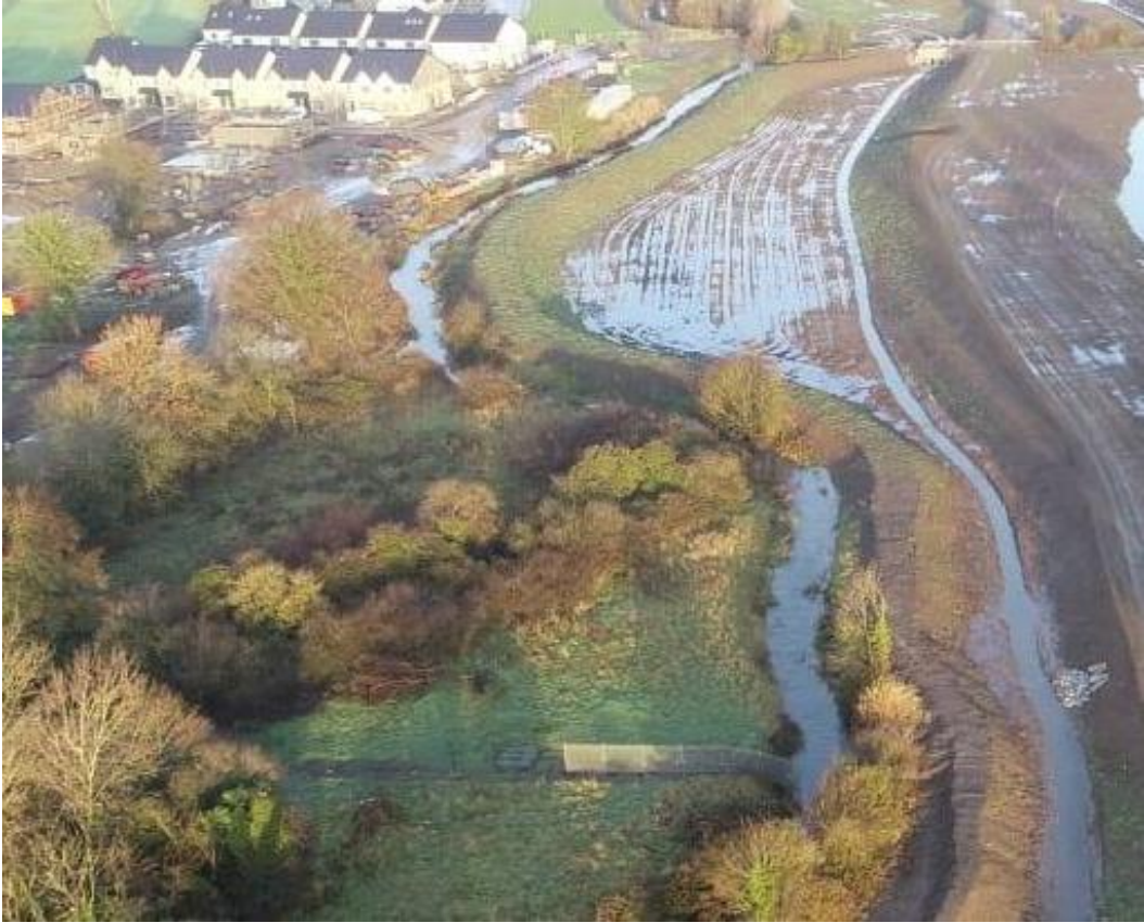
Photo 5 – Completed 'Upper Ditch' Flood Plain Works
