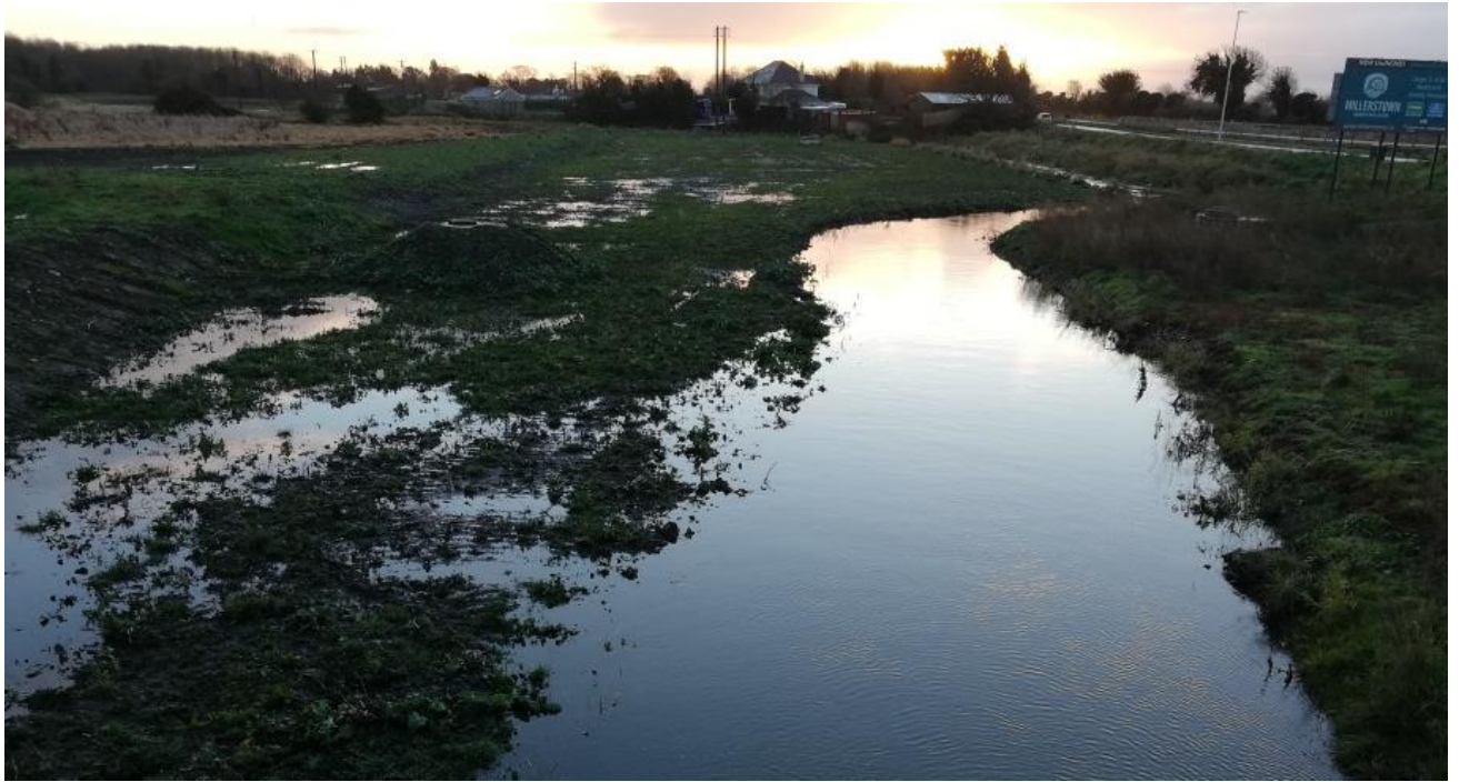
Photo 21 – Completed Lower/Rye Water Flood Plain Works
