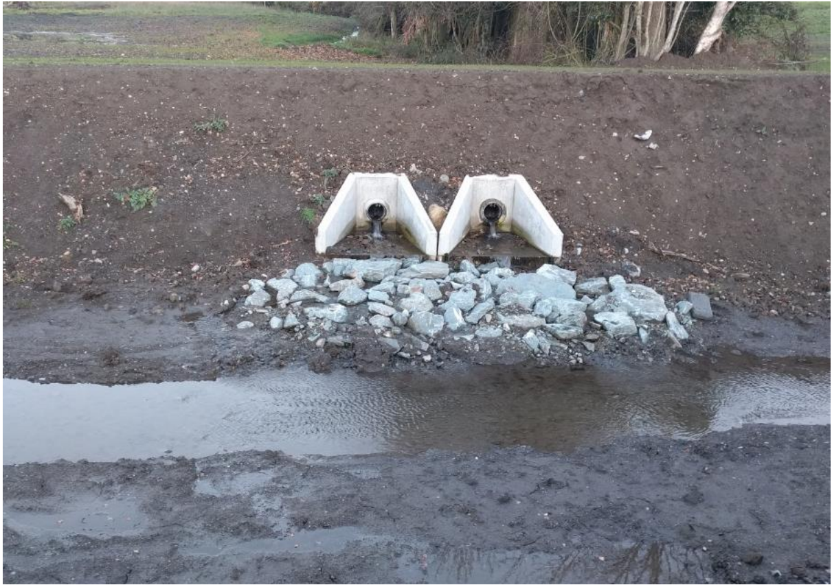
Photo 13 – Completed ‘Upper Ditch’ Flood Plain Works
