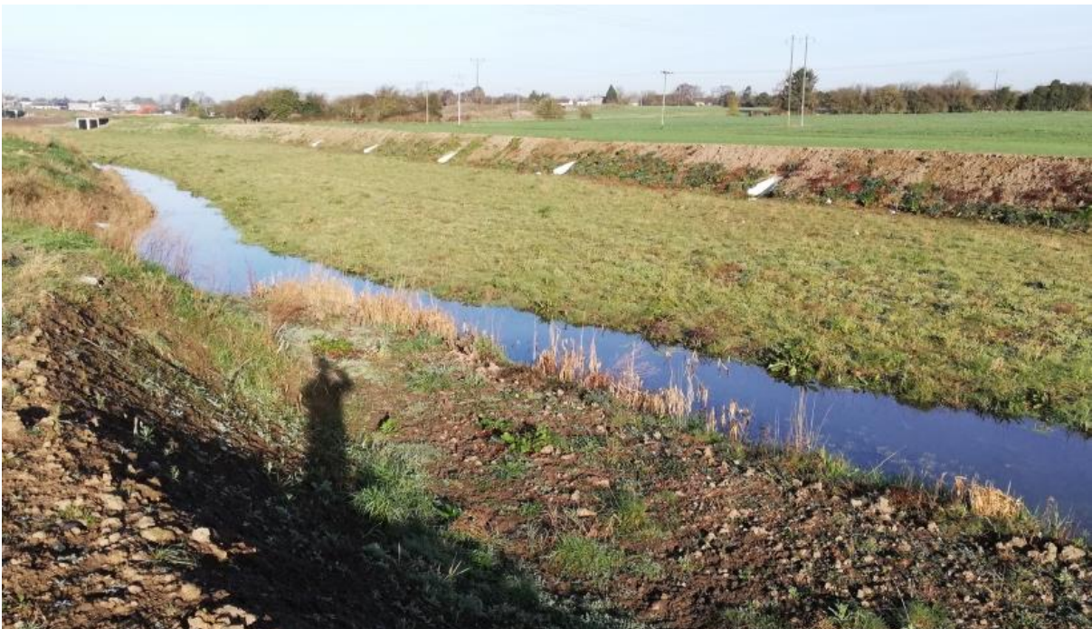
Photo 18 – Completed ‘Upper Ditch’ Flood Plain Works
