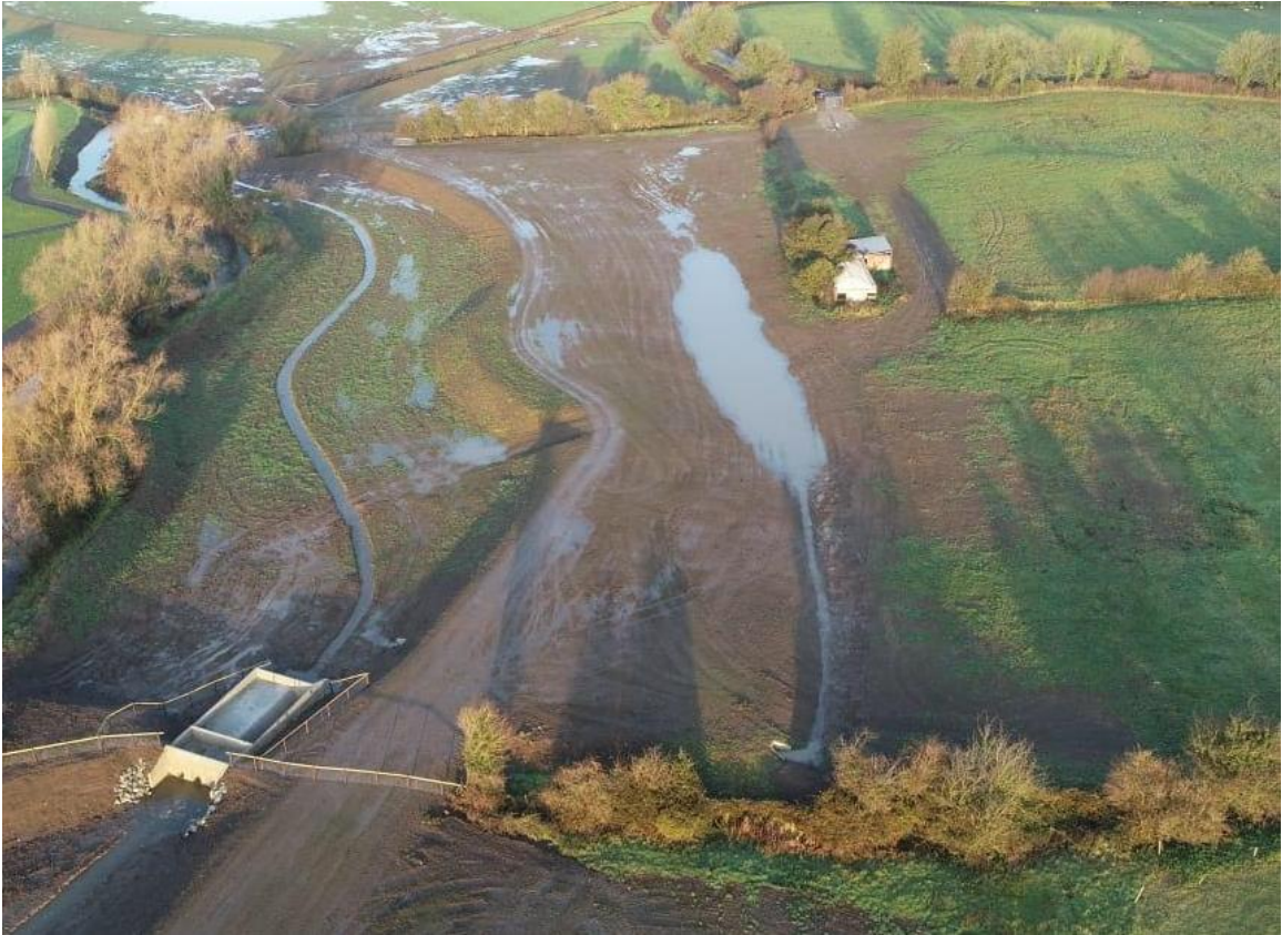
Photo 6 – Completed 'Upper Ditch' Flood Plain Works
