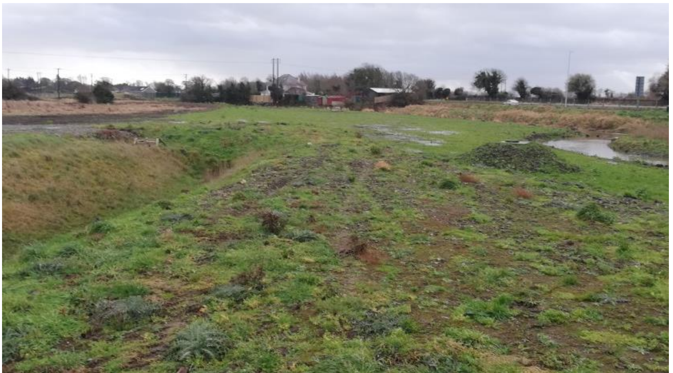
Photo 22 – Completed Lower/Rye Water Flood Plain Works
