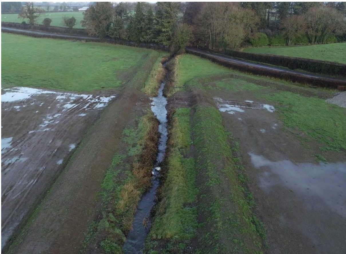
Photo 2 – Completed 'Upper Ditch' Flood Plain Works
