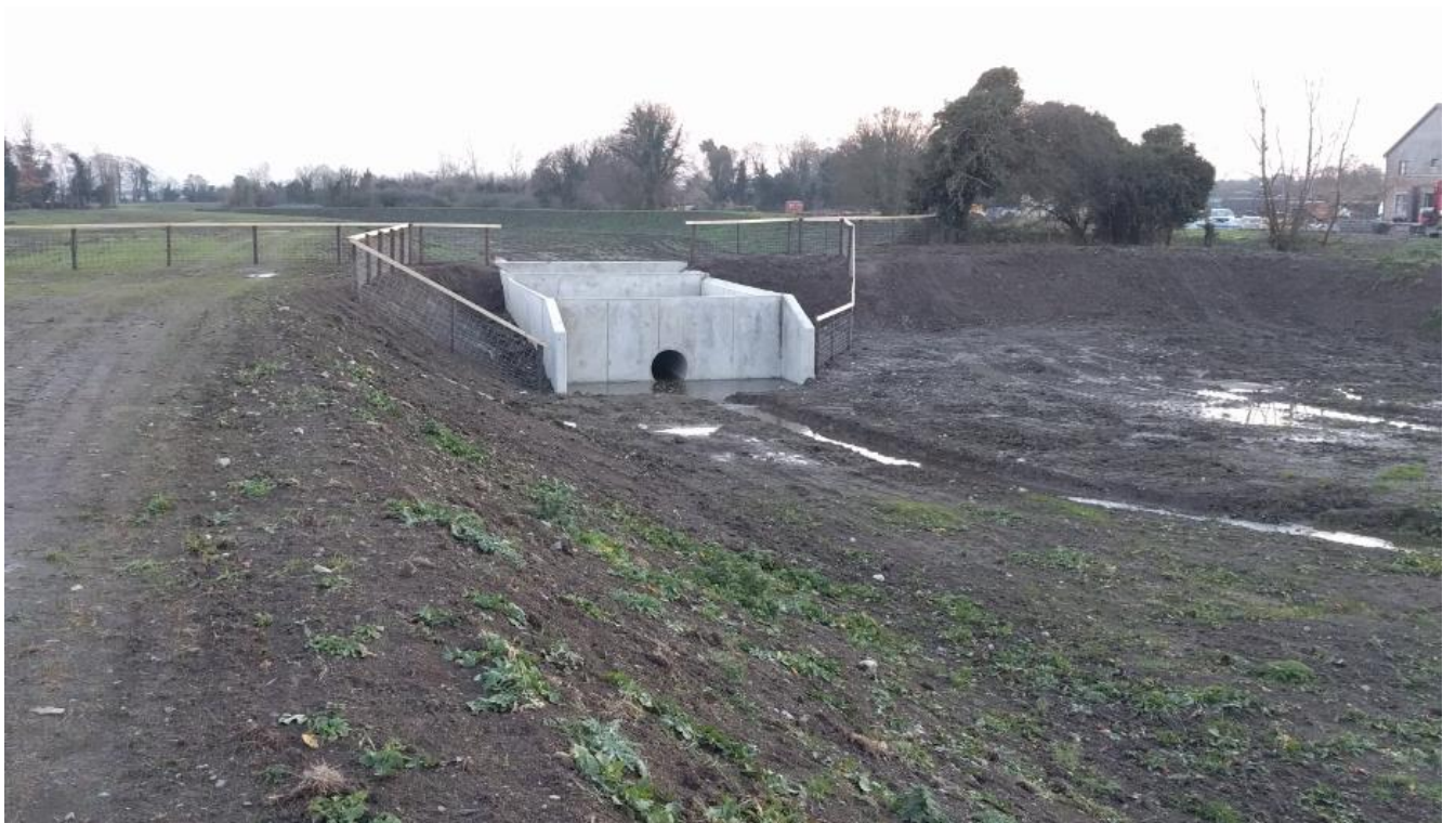
Photo 14 – Completed ‘Upper Ditch’ Flood Plain Works
