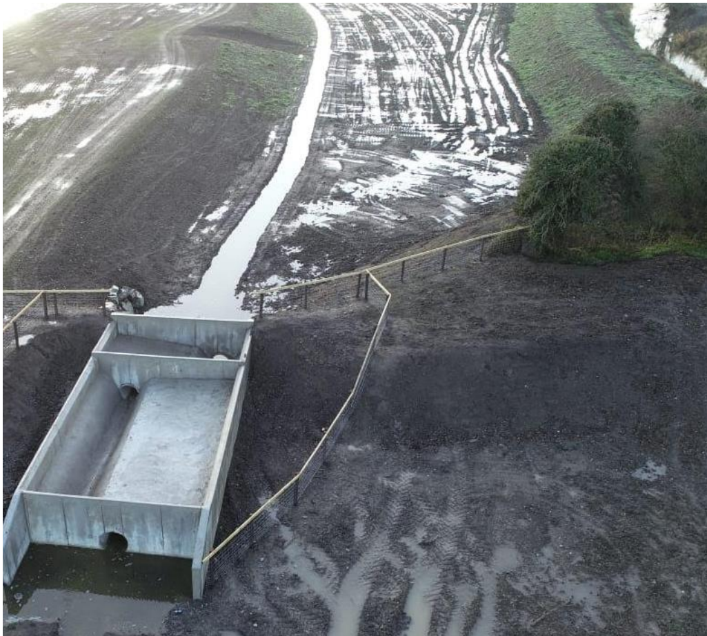
Photo 16 – Completed 'Upper Ditch' Flood Plain Works
