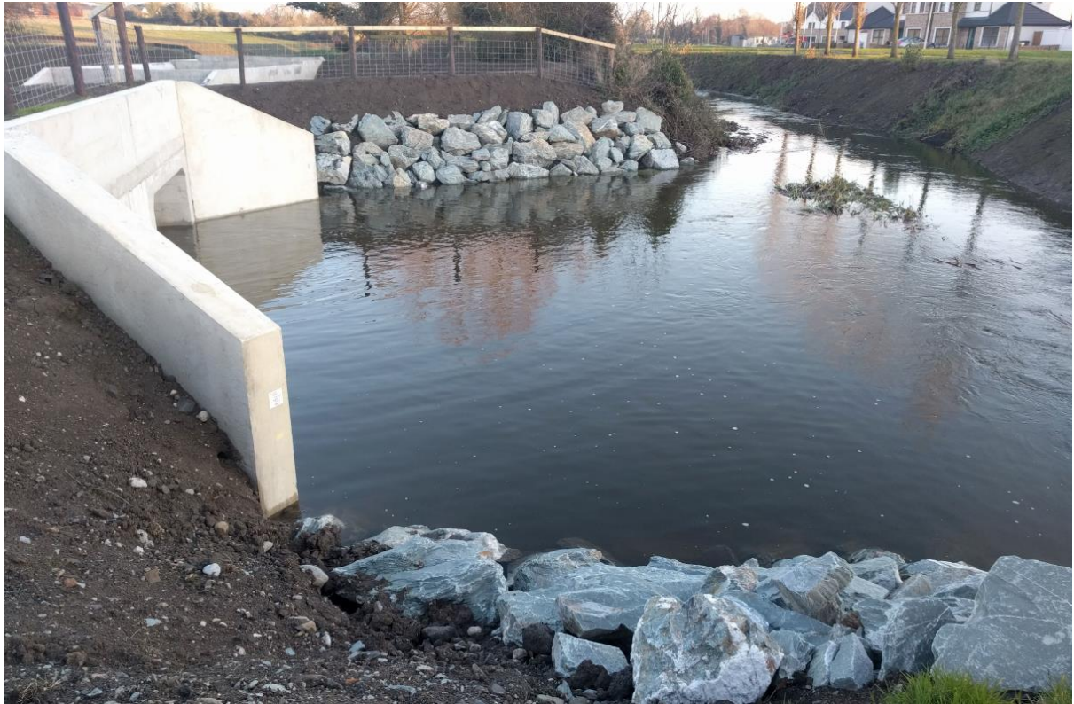
Photo 11 – Completed 'Upper Ditch' Flood Plain Works
