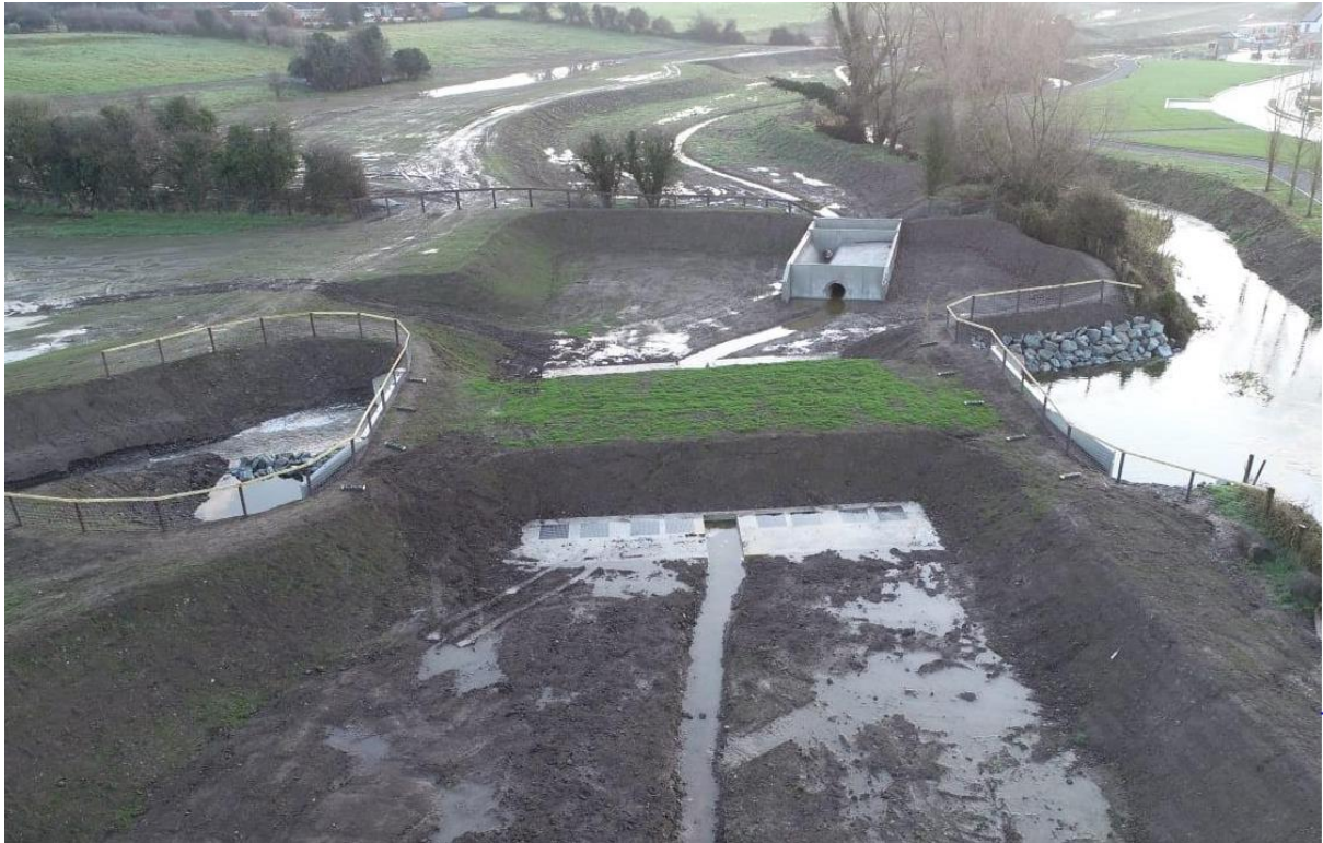
Photo 1 – Completed 'Upper Ditch' Flood Plain Works
