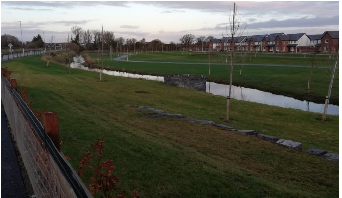
Photo 20 – Completed Lower/Rye Water Flood Plain Works
