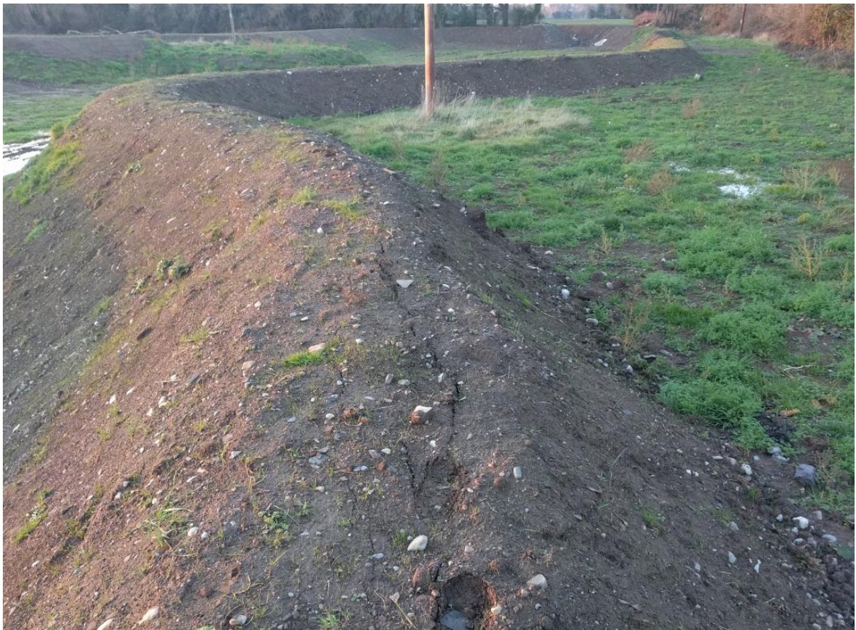
Photo 12 – Completed 'Upper Ditch' Flood Plain Works
