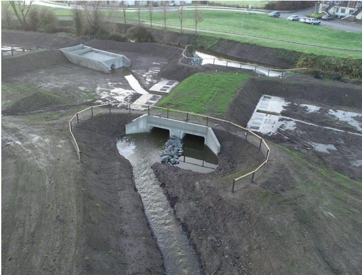
Photo 3 – Completed 'Upper Ditch' Flood Plain Works
