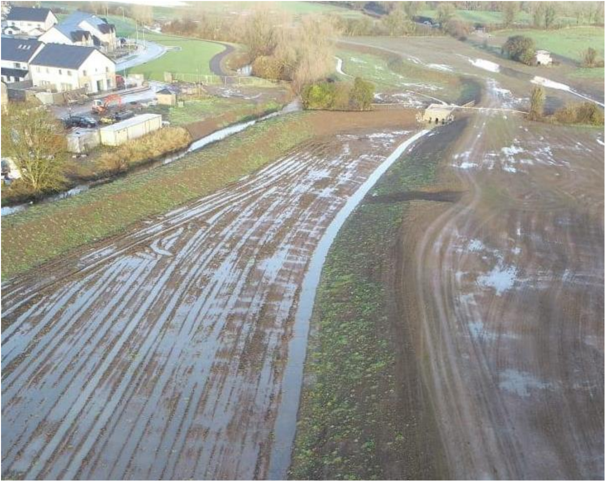
Photo 17 – Completed ‘Upper Ditch’ Flood Plain Works
