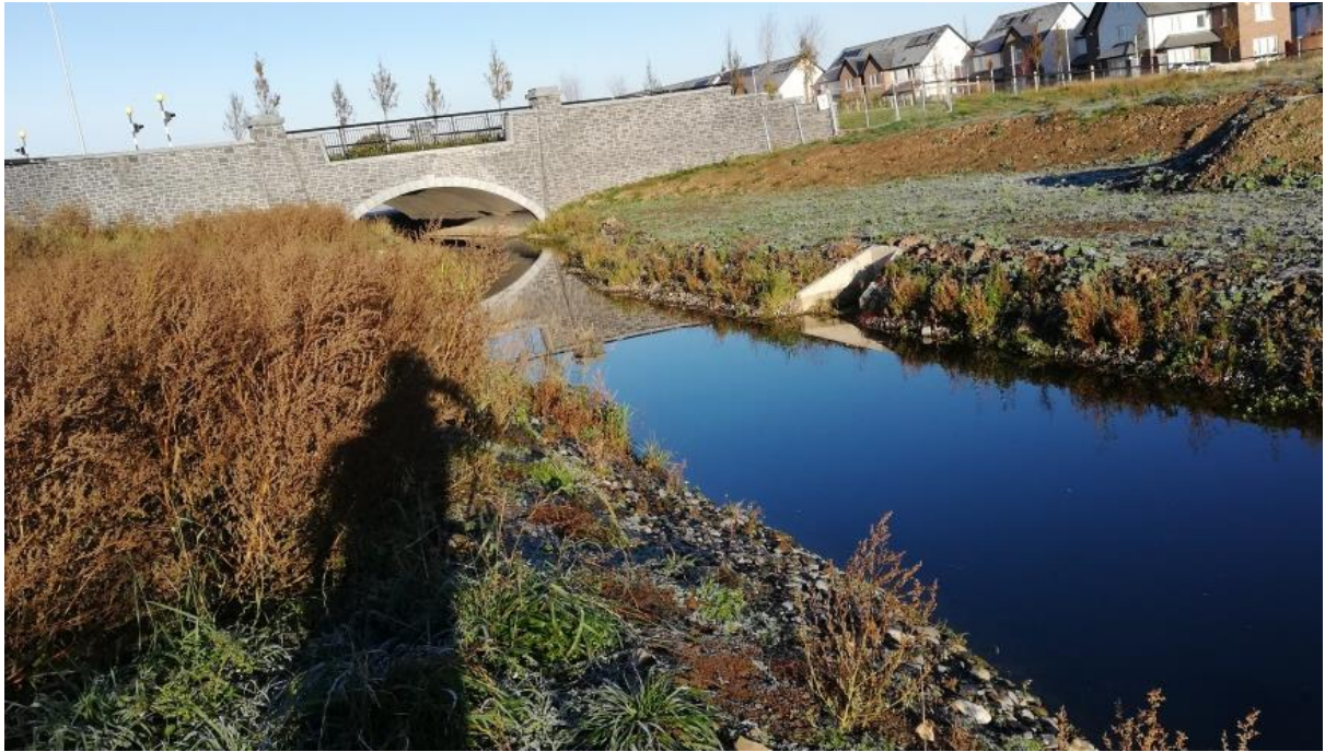
Photo 23 – Completed Lower/Rye Water Flood Plain Works
