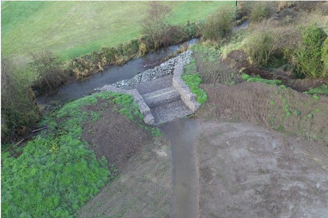
Photo 15 – Completed 'Upper Ditch' Flood Plain Works
