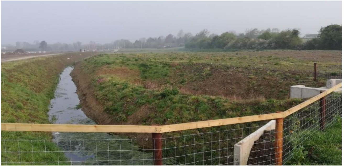
Photo 19 – Completed 'Upper Ditch' Flood Plain Works
